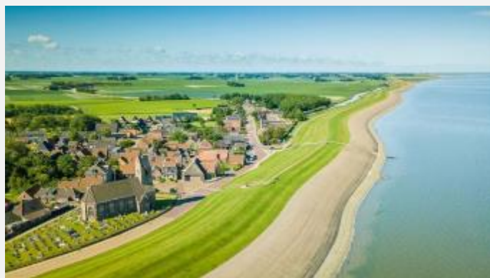
Figure 10. Coastline restoration, combining nature, coastal protection, flood risk reduction and improving biodiversity and in Fryslân (NL). Image Credit: 1DYK
